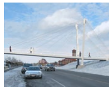
Revere Bridge (US)
