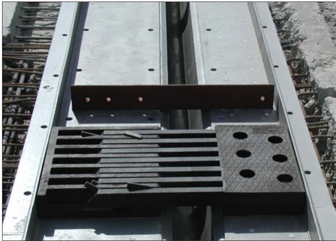
Figure 3: Anchoring of Tensa®Flex Fingers on steel substructure
