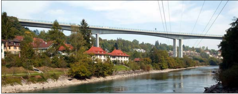
Figure 5: Felsenau Viaduct, Bern
