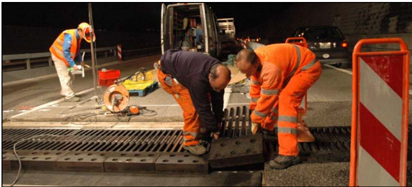
Figure 6: Nighttime Installation of the Tensa®Flex Sliding Finger at the Viaduct
