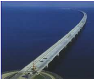
Storebælt West Bridge (Denmark) Pot bearings V_{max} = 49'000 kN Modular expansion joint type LR15 (1'200mm)
