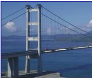
Tsing Ma Bridge (HongKong) Modular expansion joint type LR25 (max. 2'000mm)
