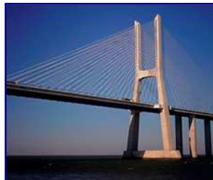
Vasco da Gama Bridge (Portugal) Pot bearings V_{max} = 39'000 kN Modular expansion joint type LR9 (720mm)
