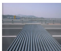
Modular expansion joints
