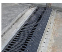
Sliding finger joints
