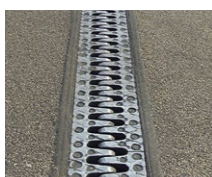
Cantilever finger joints
