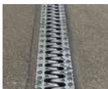
Cantilever finger joint
