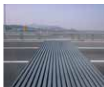
Modular expansion joints
