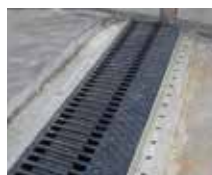
Sliding finger joints
