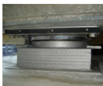
Spherical bearings
